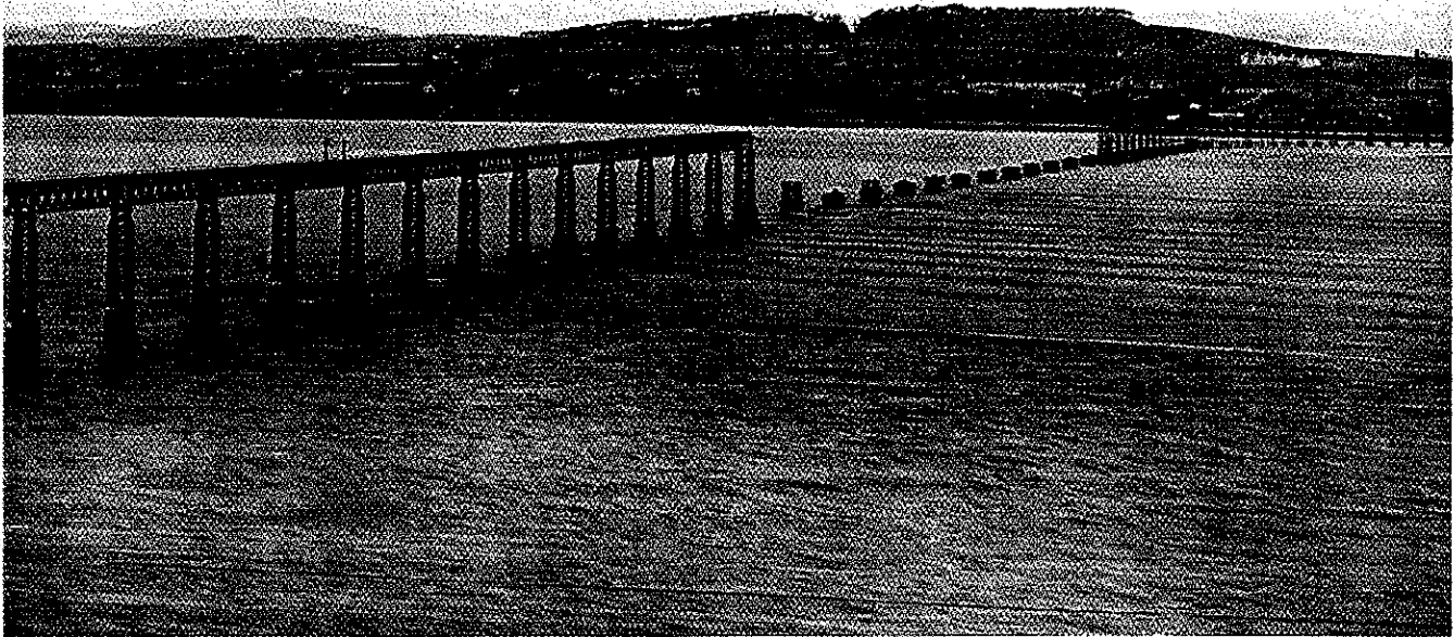
Fig. 4. Tay rail bridge after 1878 collapse (viewed from south)
